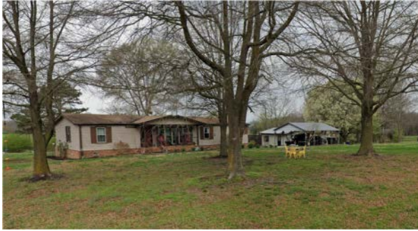
VIEW OF RESIDENCE IN NEIGHBORHOOD
