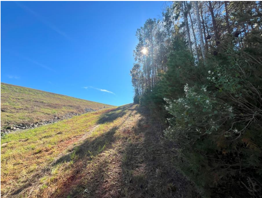
Photo 50. Field map number 13 facing South with the drainage ditch.
