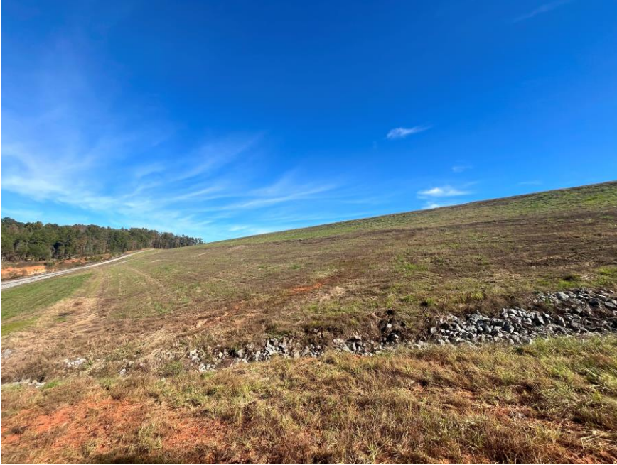
Photo 51. Field map number 13 facing East towards the CRWTP parcel. The rocks make up a drainage ditch.
