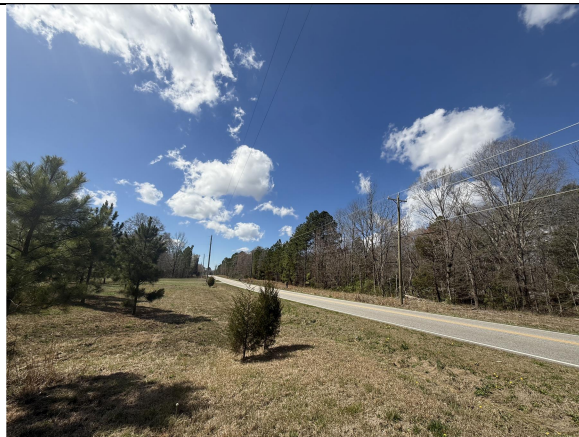
Highway View – Westbound Direction
